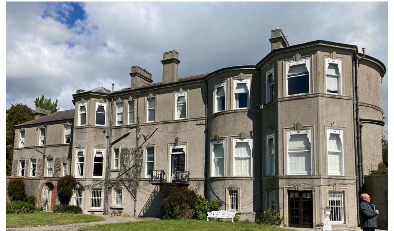
Dalguise House - Existing
